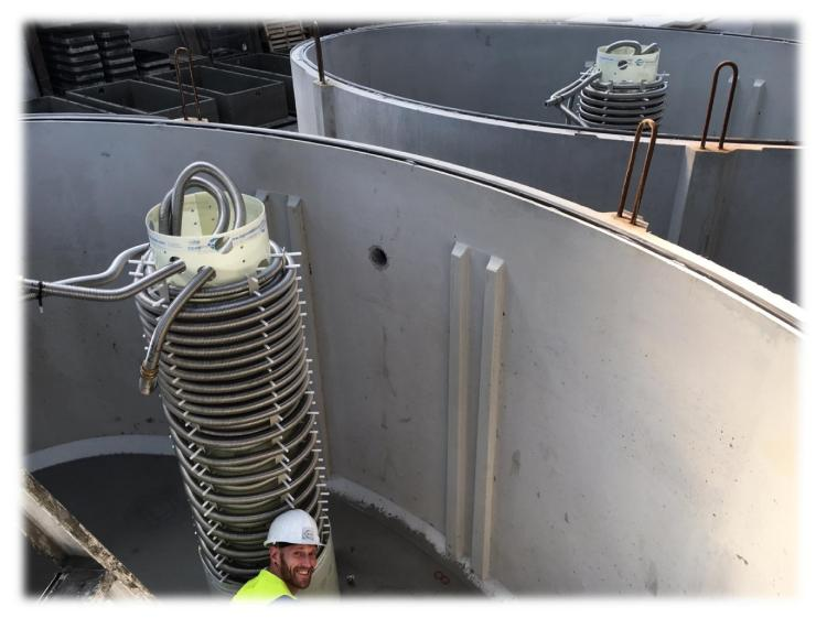
Two concrete rainwater tanks of each 20.000 Liter are equipped with a vertical heat exchange system. This system is made out of stainless steel and polyester because of the possible high temperatures. The concrete tank is made out of high quality C35/45 concrete.
