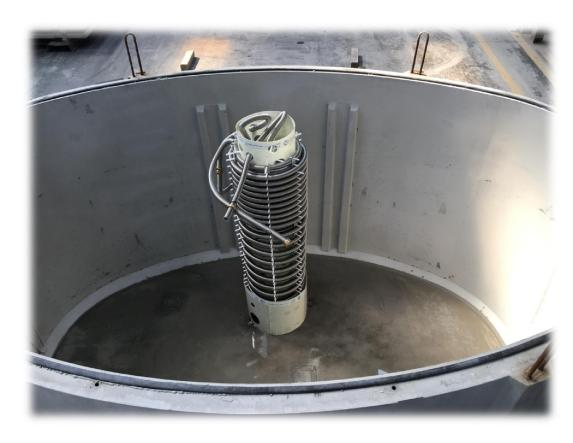
Each heat exchange system consists out of 2 stainless steel tubes with a surface of approx. 9 m2 per piece. This means a total of 18 m2 per rainwater tank. The two tanks are equipped with a high and low connection in order to make use of the temperature difference between the bottom and the top of the tank.
