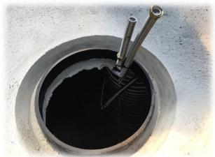
The tanks are equipped with a class D cover for heavy traffic and a manhole of 600 mm. The connections on the tanks are equipped with a rubber gasket which allows the coupling of the two tanks, these interconnections are placed at several levels to use heat differences at different water levels. The connections of the heat exchange systems are placed at the top of the tank. Two connections per tank with a 6/4" connection.
